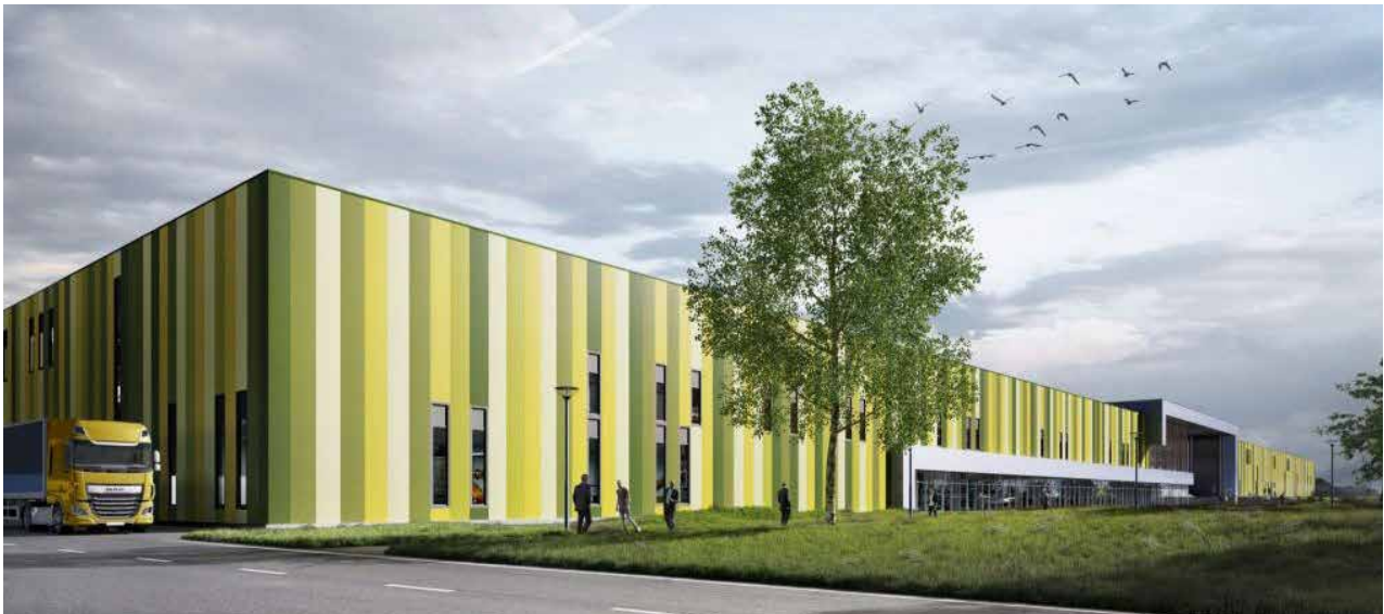
Figure 38 Brainport Industries Eindhoven building
